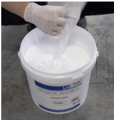
Immergere il nastro in colla vinilica Link Glue V20 Drop the tape inside the basket of Link Glue V20
